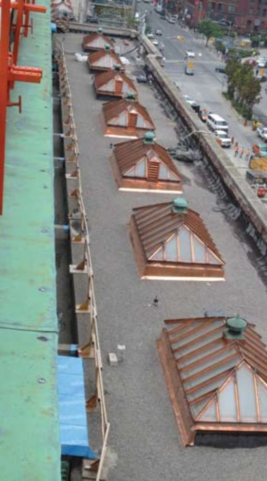
New skylights along the Front Street wing of the Station.
