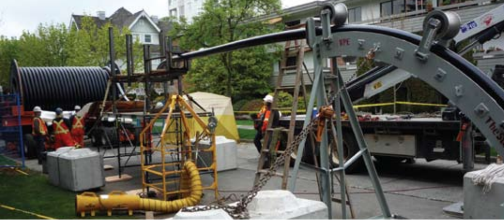
Cable being pulled from a reel into a cable vault.
