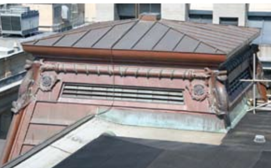
One of the four complex corner sections.
