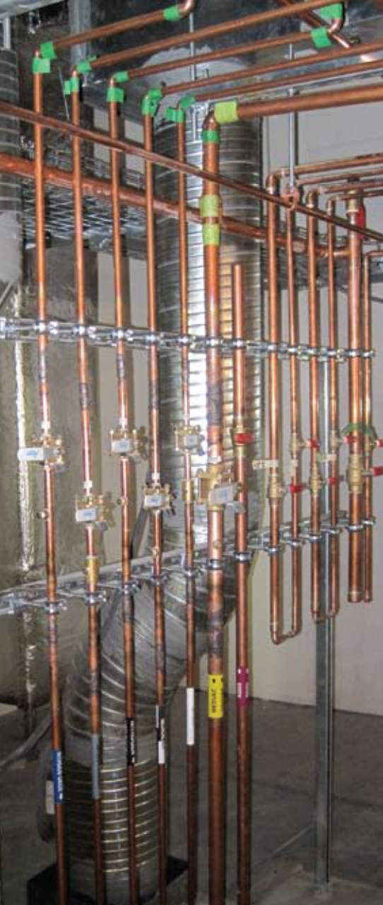
A "pipe rack" station in the interstitial area between patient floors showing the soldered domestic water lines and the taped, ready-to-be-brazed medical gas lines.
