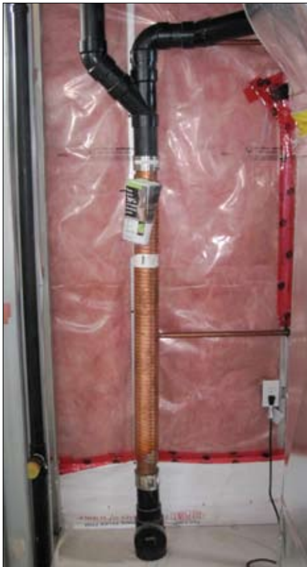
The copper Drain Water Heat Recovery Unit on the main drainage stack captures heat from warm or hot waste water which is used to pre-heat incoming water.
