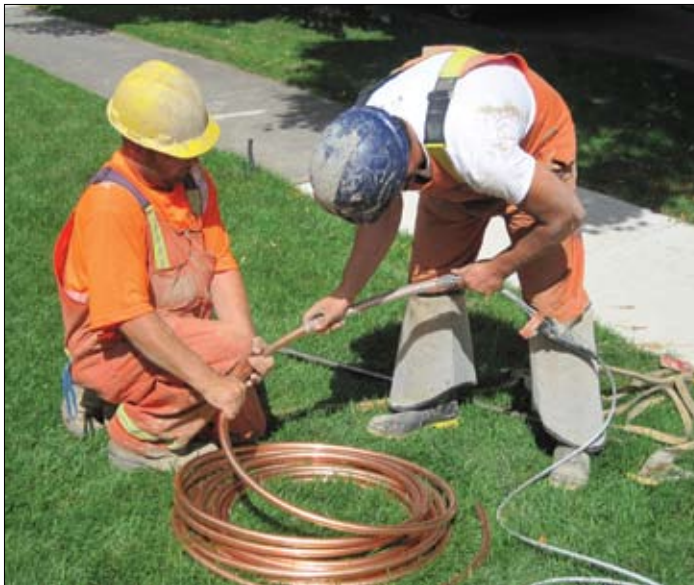
The cable and torpedo splitter are attached to the Type K copper water tube.
