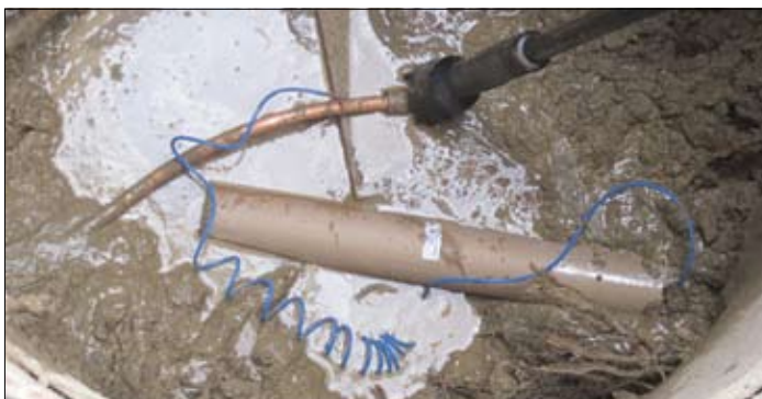
The completed replacement at the curb stop includes a 5.5 kg (12 lb) sacrificial zinc anode.
