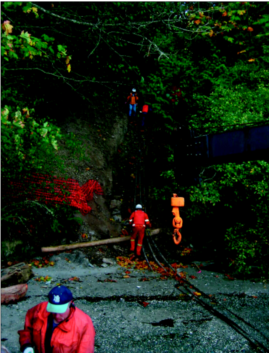
Removal of the existing 30-year old cable.
