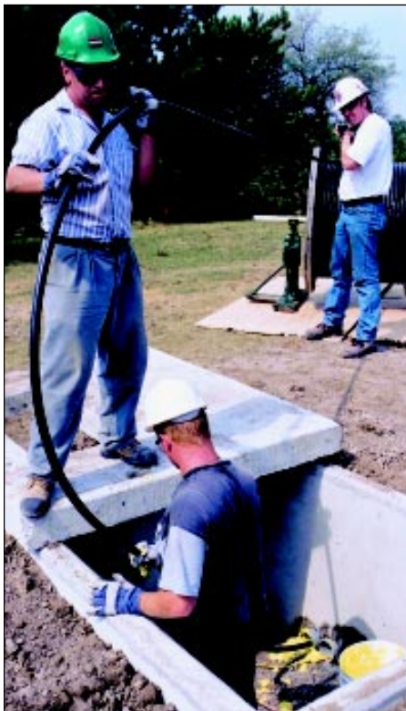
One of three 15 kV #1/0 AWG copper cables being installed in an underground conduit to bring power from the wind turbine to the grid.
