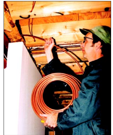
Lightweight copper tube is easily installed between joists.
