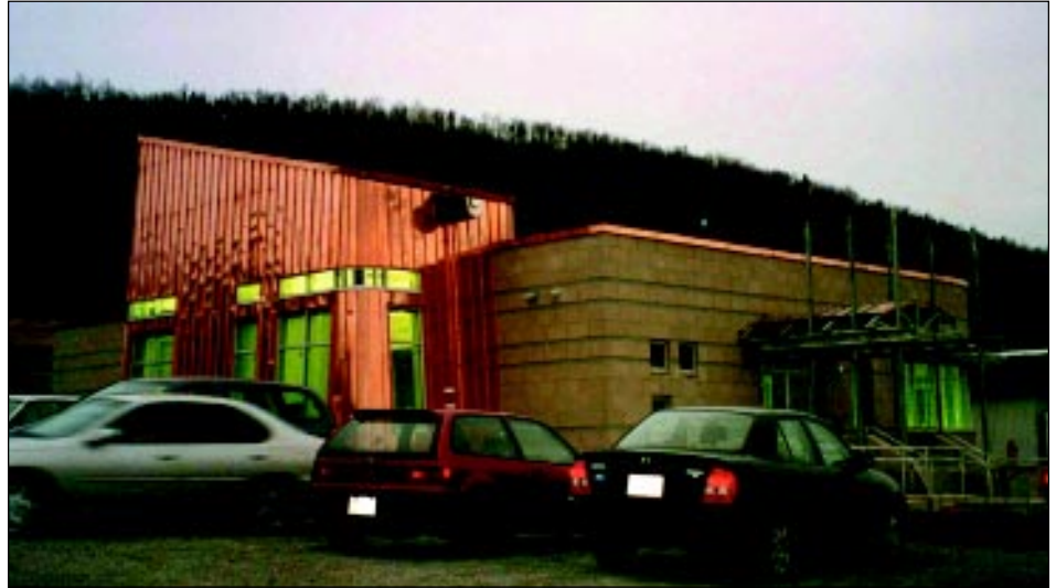
Copper cladding was used to emphasize sections of the Detachment.
