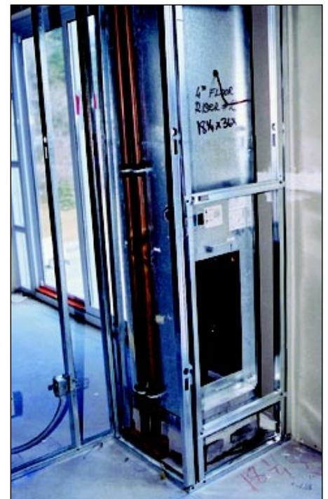
*Hot water supply and return lines below the mechanical room on the top floor of No. 10 Old York Mills.*
