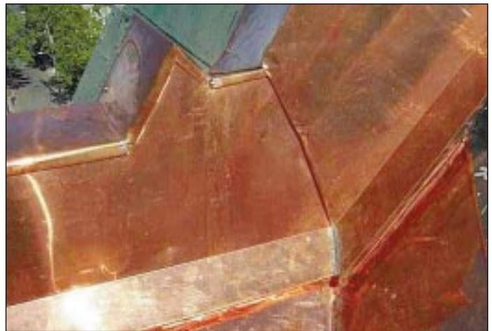
sheet copper was installed over a plywood substrate, with a membrane and building paper underlayment. The 65,000 lbs. of copper was supplied by Canadian Brass & Copper of Concord, Ontario.
