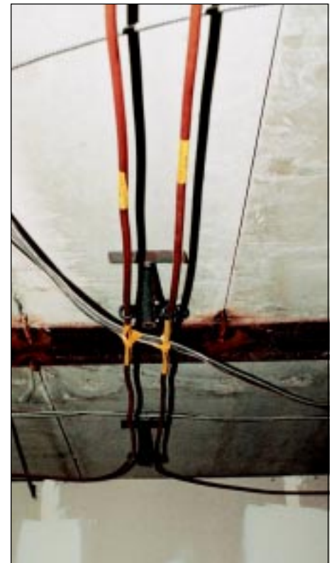
A clever bracket system made installation of the copper tube easier in the corridors.
