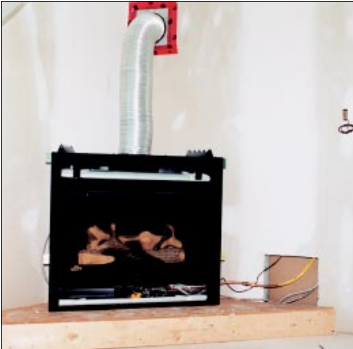
A corner gas fireplace with the copper supply line before installation of the mantel.
