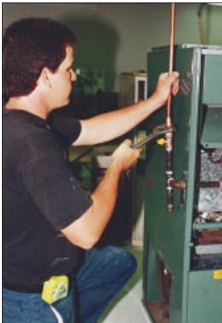
Installation of a copper supply line to a furnace.
