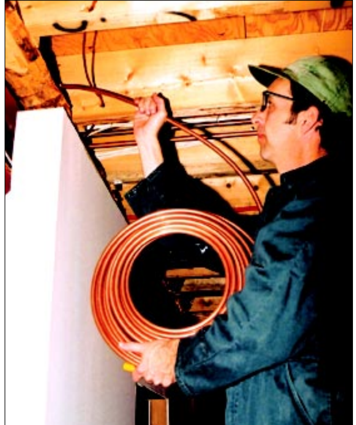
Lightweight Type G/GAS copper tube is easily installed between joists.
