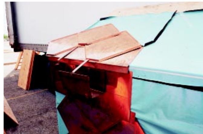
Left: Mock-up of prefabricated copper shingle roof, cladding, and gutter system, St. Justin's Church, London, Ontario.
