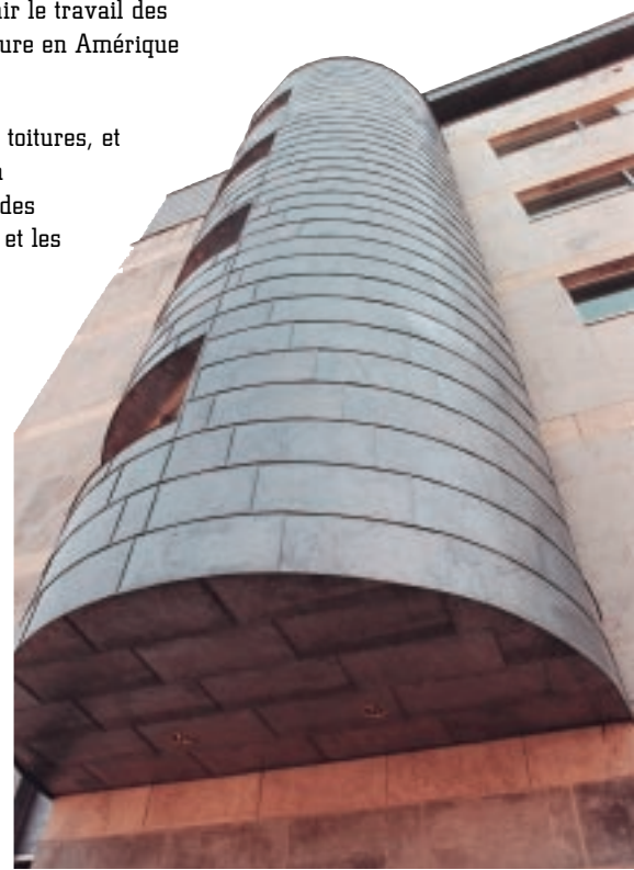
Left: Example of mill-produced, prepatinated copper, with striking resemblance to naturally aged copper.
